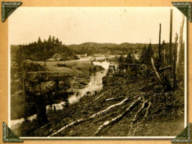
Upstream view of High Falls dam in its early days
