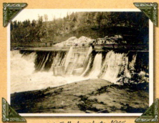
High Falls log chute, 1905
