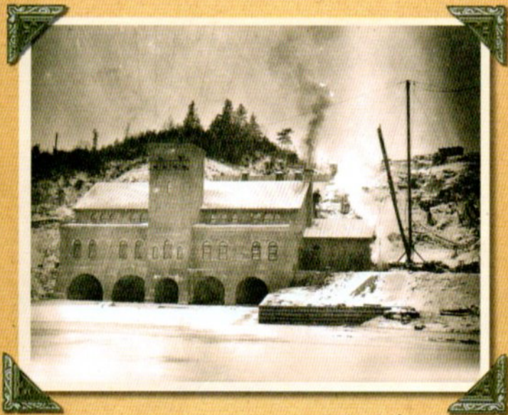
Winter at High Falls Dam and Power House
